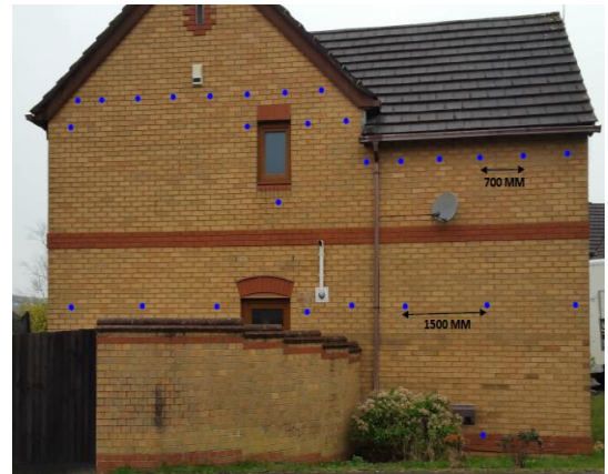
Conventional Bead Drill Pattern
